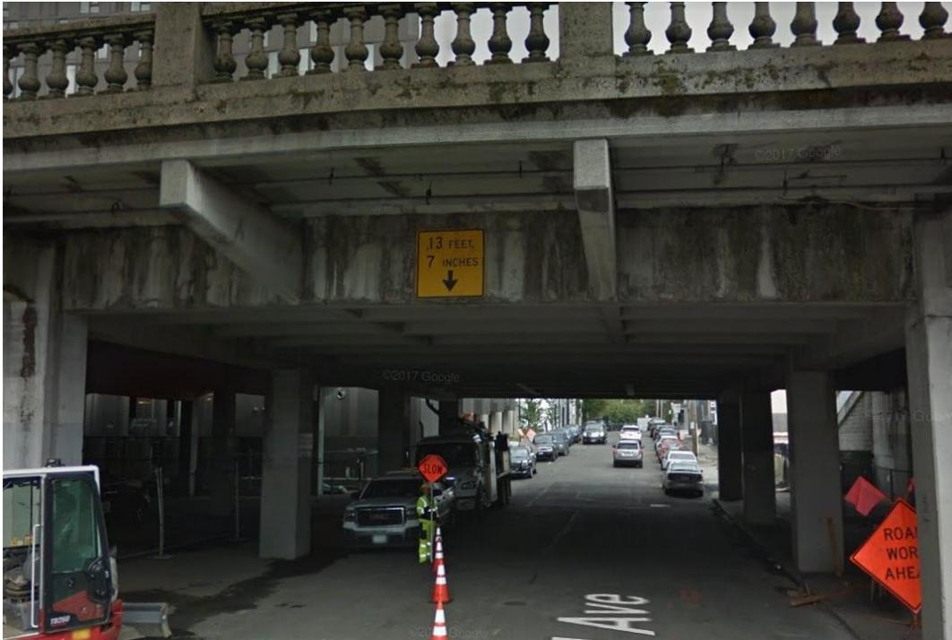
Figure 7. Looking north at limited vertical clearance over NE/SE 3rd Avenue
