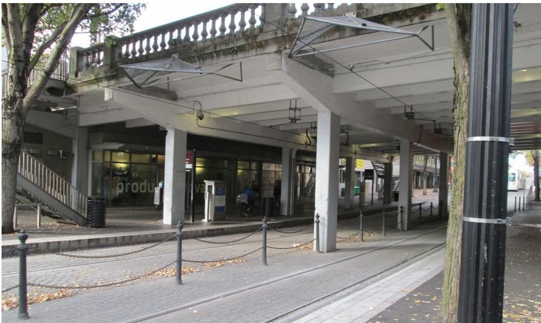
Figure 8. Looking north at limited vertical clearance over TriMet MAX Light Rail on NW/SW 1st Avenue
