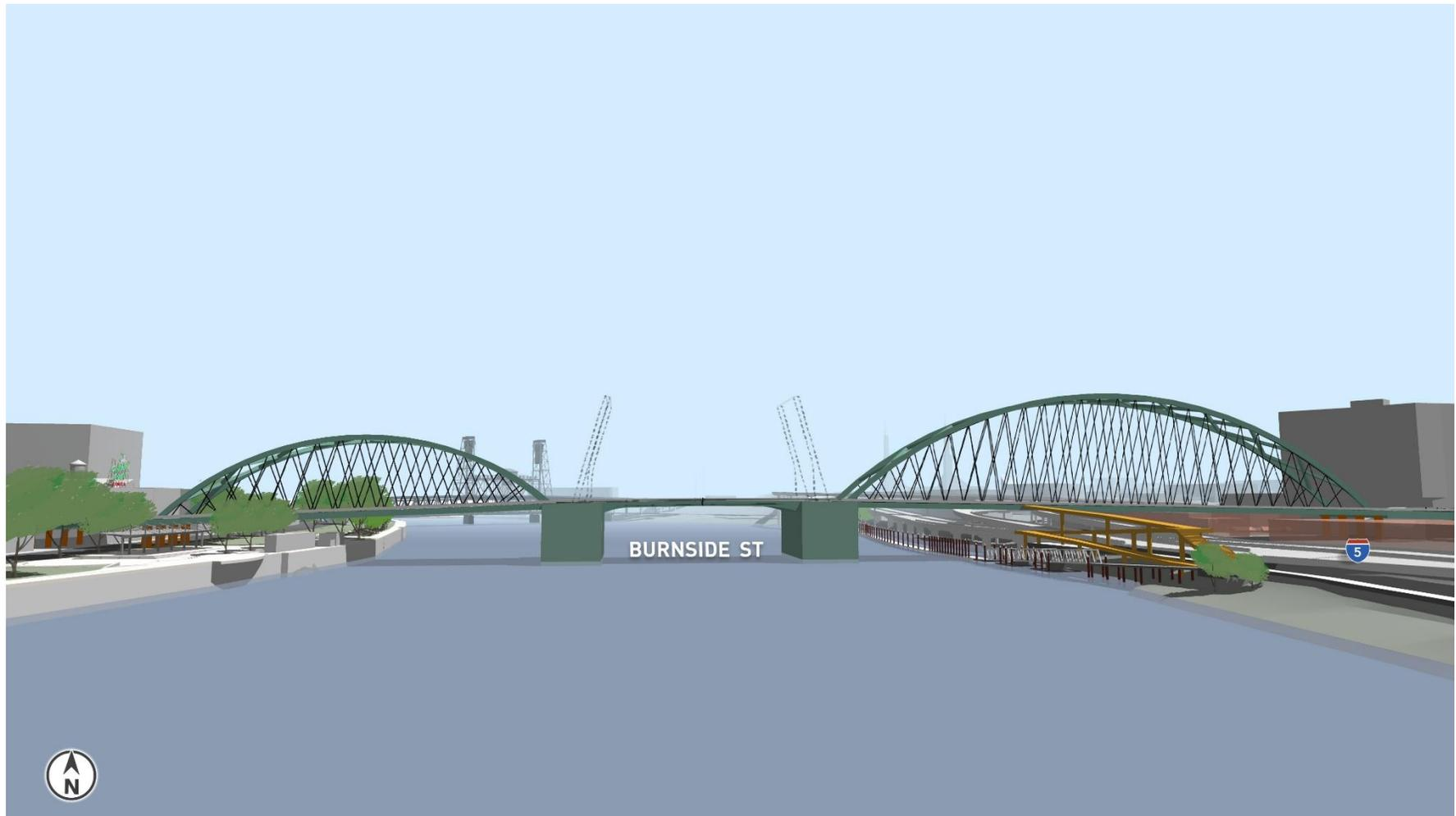
Figure 19. Replacement Alternative with Long-Span Approach – Profile (Lift)
