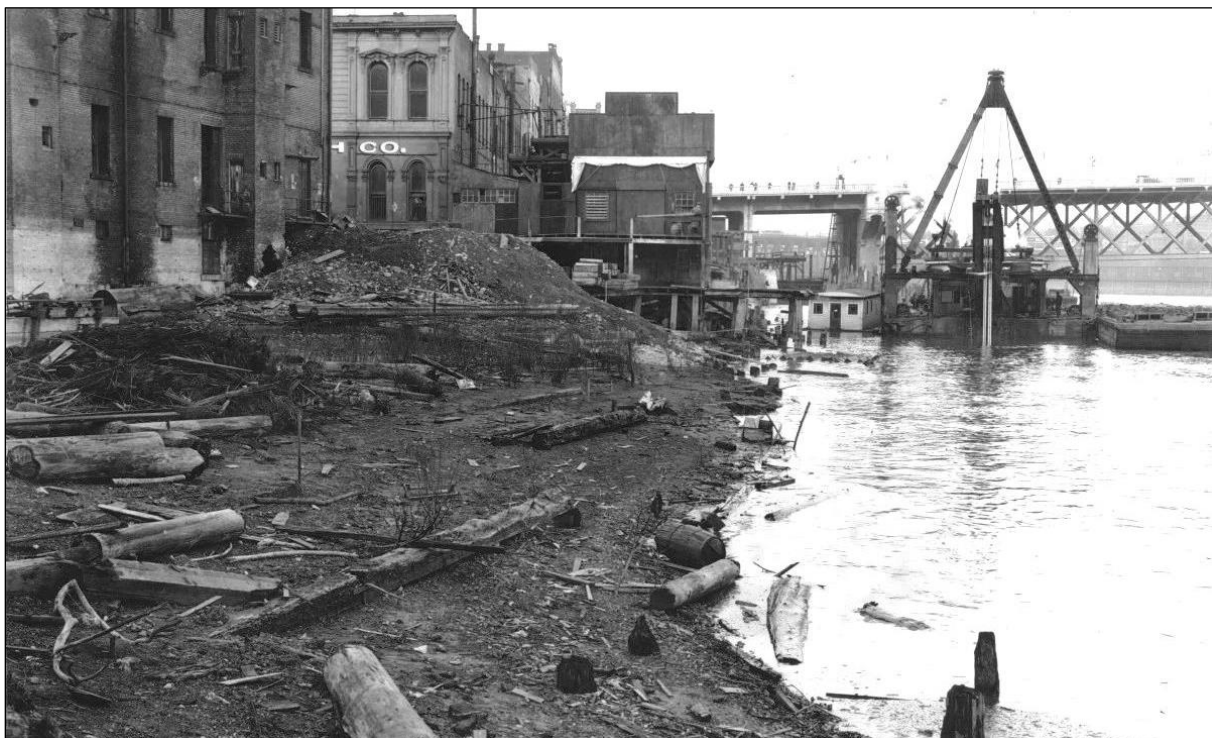
Figure 5-31. Clearance of docks and wharves in preparation of construction of the Harbor Wall, with the Burnside Bridge to the north. Photo dated January 31, 1928.
