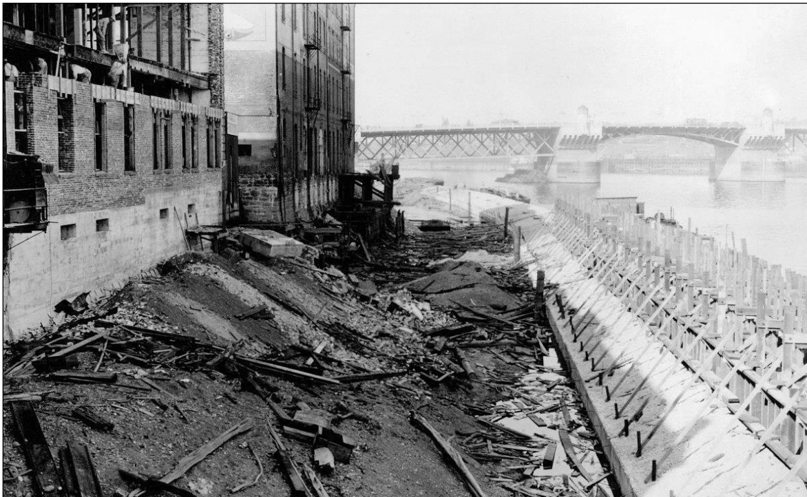
Figure 5-37. Construction in progress of Harbor Wall forms with view of debris on shoreline and reconstruction of rear wall of building damaged during dock removal on September 28, 1928.
