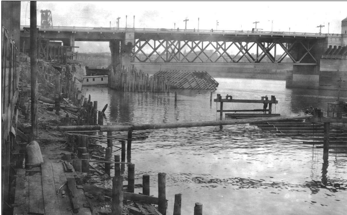
Figure 5-32. Dock remnants with continuing demolition in preparation of construction of the Harbor Wall, with the Burnside Bridge to the north. Photo dated March 8, 1928.
