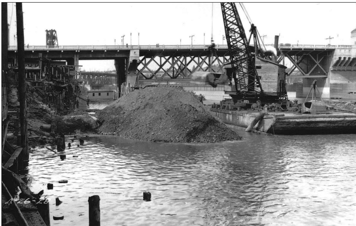
Figure 5-33. Stockpiling of dredged Harbor Wall fill immediately above the Burnside Bridge. Photo dated April 26, 1928.
