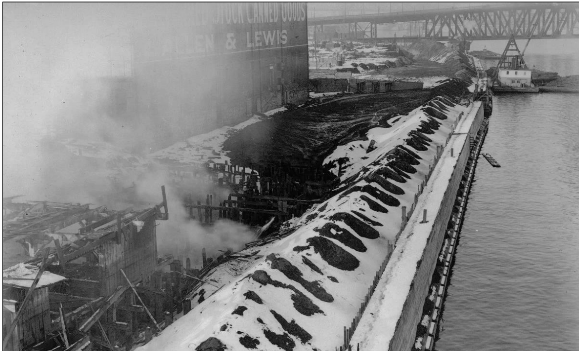
Figure 5-29. Remnant of docks and placement of Harbor Wall fill at the Allen & Lewis warehouse, looking downriver. Compare with Figure 5-27 and Figure 5-28. Photo dated February 5, 1929.
