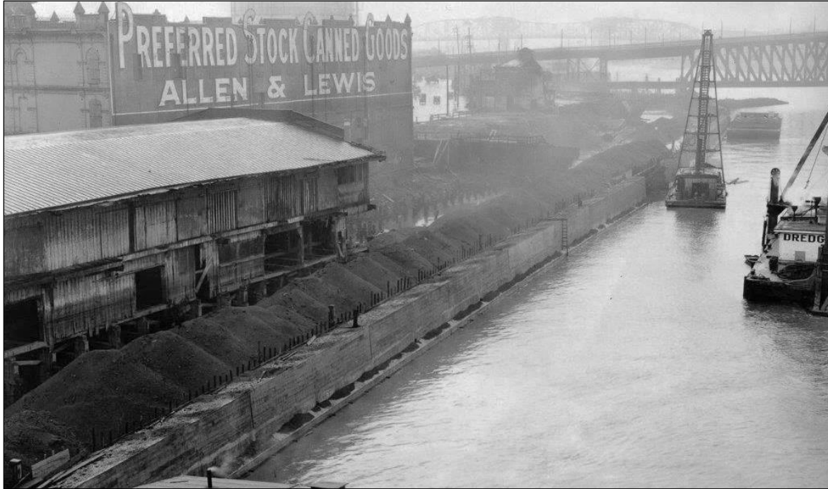
Figure 5-28. Remaining dock and Harbor Wall construction with placement of fill at the Allen & Lewis warehouse, looking downriver. Note the Gillen-Cole building is gone and the Portland Gas Manufacturing Purifying House to the north is partially razed. Compare with Figure 5-29. Photo dates December 23, 1928.
