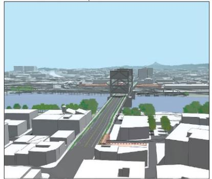
Long-span Alternative / Through-truss / Bascule
