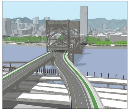
Long-span Alternative / Through-truss / Bascule
